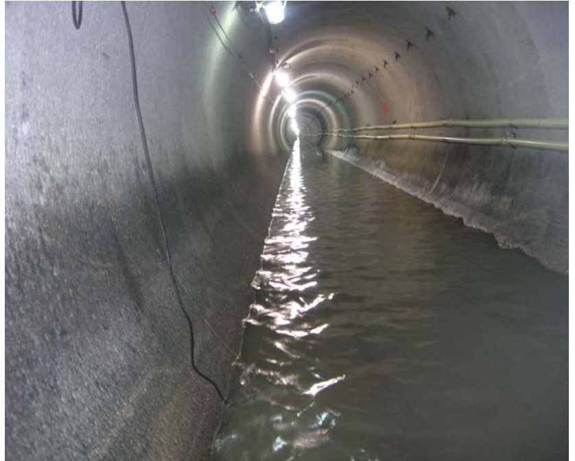
Photo of the tunnel dug by Mole Constructors in Gwinnet County, Georgia.
