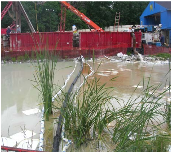
Three tanks make up the system and involve the use of Floc Logs and particle curtains to treat incoming water and remove sediments before discharge.
